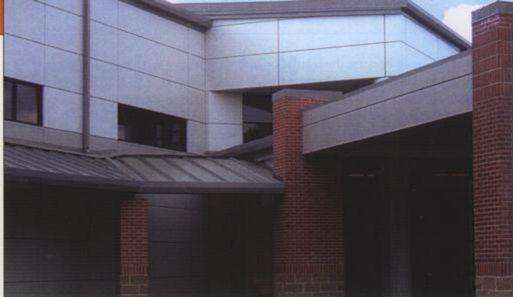
The new Sheridan Elementary School in Sheridan, AR, now features a modern metal facade with CENTRIA's Formawall Dimension Series metal wall panels.
